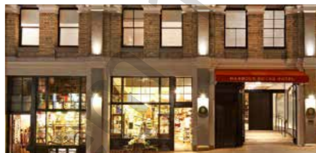
Shop Front Display, wall lights The Rocks Hotel, Sydney
